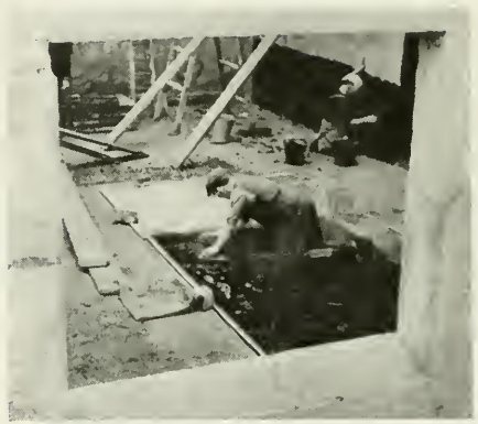
Application of asphalt damp-proofing
